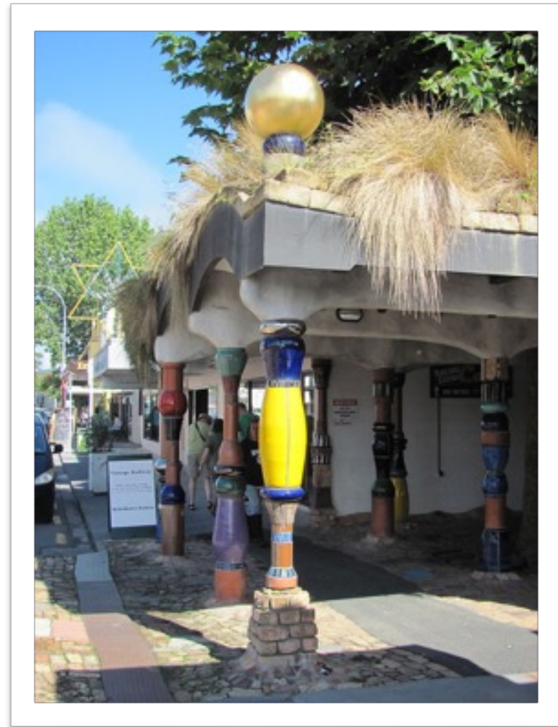
Public Toilets in Kawakawa New Zealand. Photo by Reinhard Dietrich "Hundertwasser-WCaussen"- Wikimedia Commons
